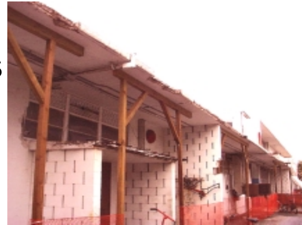
Collapsing Aviation Facility at KMR Where safety fencing is required to protect personnel from falling debris and cave in
